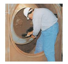
**CERAMIC REBUILD PUTTY** Highly advanced epoxy putty that provides suitably treated equipment with exceptional resistance to erosion, cavitation, corrosion and chemical attack. Repair or rebuild pumps, impellors, liners, valves, elbows and other components used in power plants, pulp and paper mills, and other industrial applications.
